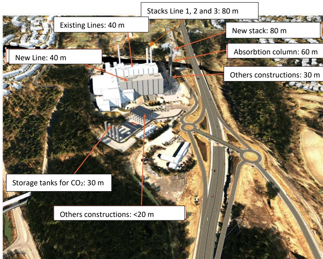
Figure 5 Klemetsrud WtE plant with carbon capture; stacks and building heights used in the model. Building for «new Line» is not included in the model
